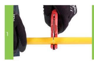
With a set of pipe cutters /shears cut the pipe at 90° ensuring the pipe is square on the end.
