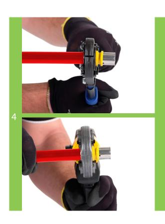
Proceed to crimp the fitting until jaws of tool are completely closed.
