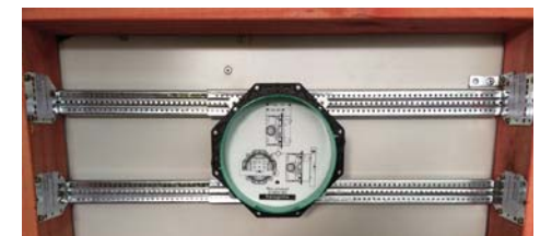
A Hansgrohe iBox shower valve installed using BK4 brackets.
