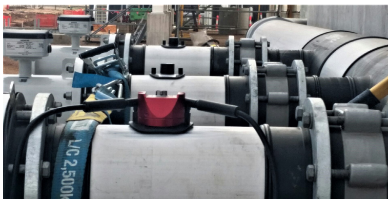
More than eighty sensor points were to be joined to pipes ranging in size from 225mm to 630mm. Due to the compact nature, several sensors were often designed to be installed circumferentially around the pipe.
