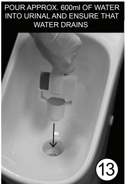
INSERT NEW BIO-FRESH AND LOCATE ONTO BIO-SEAL
