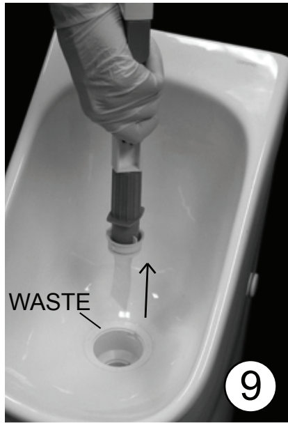
PULL TOOL UP TO EXPOSE BIO-SEAL. POUR WATER INTO URINAL TO CLEAN PLASTIC WASTE
