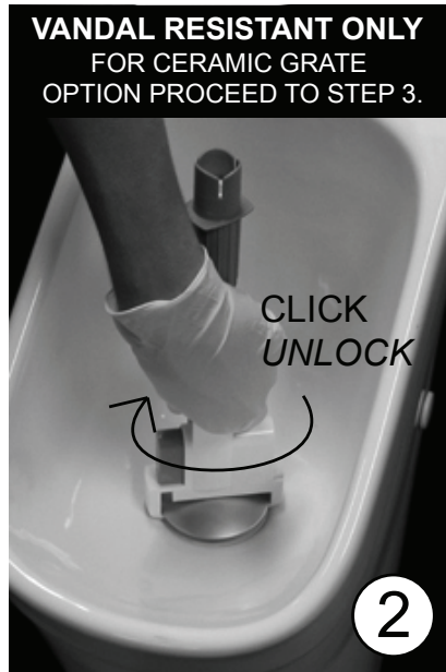
RELEASE BUTTON AND ROTATE TOOL CLOCKWISE TO UNLOCK GRATE
