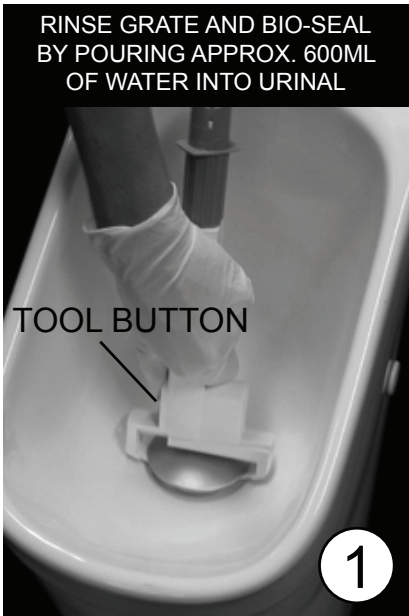
PRESS TOOL BUTTON AND SLIDE PRONGS UNDER GRATE
