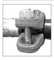
Assemble the joint by inserting the grooved end of the sprinkler piping into the opening of the coupling. The grooved sprinkler piping shall be inserted into the coupling until contact with the center leg of the gasket occurs. A visual check is required to verify that the coupling keys align with the groove in the sprinkler piping and engage with the spacer on the inlet end of the flexible hose.
