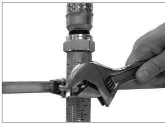
2b. FOR STYLES AB1 AND AB10 BRACKETS ONLY: Close the center gate assembly around the sprinkler reducing nipple. Swing the pivot screw and washer into the slot on the gate, and tighten the wing nut to a torque of 50 inch-lbs/6 N•m (approximately hand-tight, plus ½ to ¾ of a turn). NOTE: Verify that the washer is seated under the head of the wing nut.
