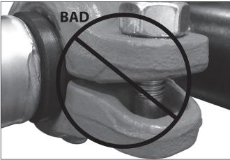
6. Visually inspect the bolt pads at each joint to verify that metalto-metal contact is achieved, in accordance with step 5.
