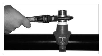
Apply pipe joint compound or PTFE thread sealant tape to the tapered threads of the adapter nipple, in accordance with the pipe joint compound or tape manufacturer's instructions. Using a pipe wrench, tighten the adapter nipple into the sprinkler piping.
