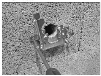
2. Place the Style AB3 Bracket over the hole cut into the wall or ceiling in Step 1. Secure the Style AB3 Bracket to the wall or ceiling using ¼-inch/6-mm diameter screws through each of the mounting holes on each side of the bracket. Tighten the two screws compeltely until the bracket is retained firnly against the wall or ceiling. NOTE: The selected screws must be appropriate for the wall or ceiling material. Refer to the hardware manufacturer's instructions for each application.
