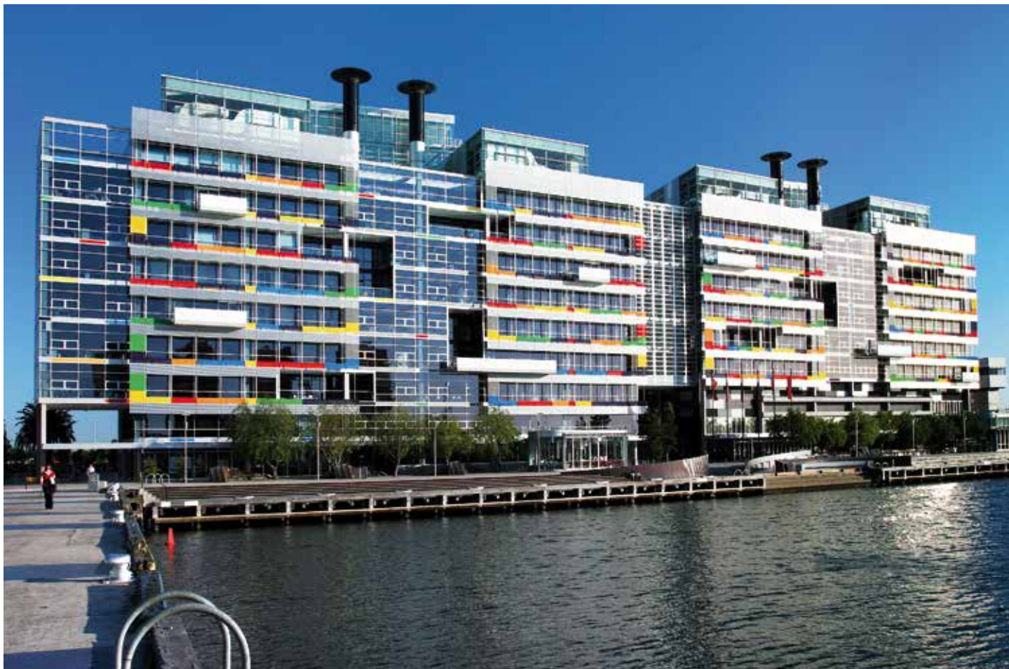
Zip Touch-Free washroom systems are a feature of the National Australia Bank, Docklands, Melbourne.
